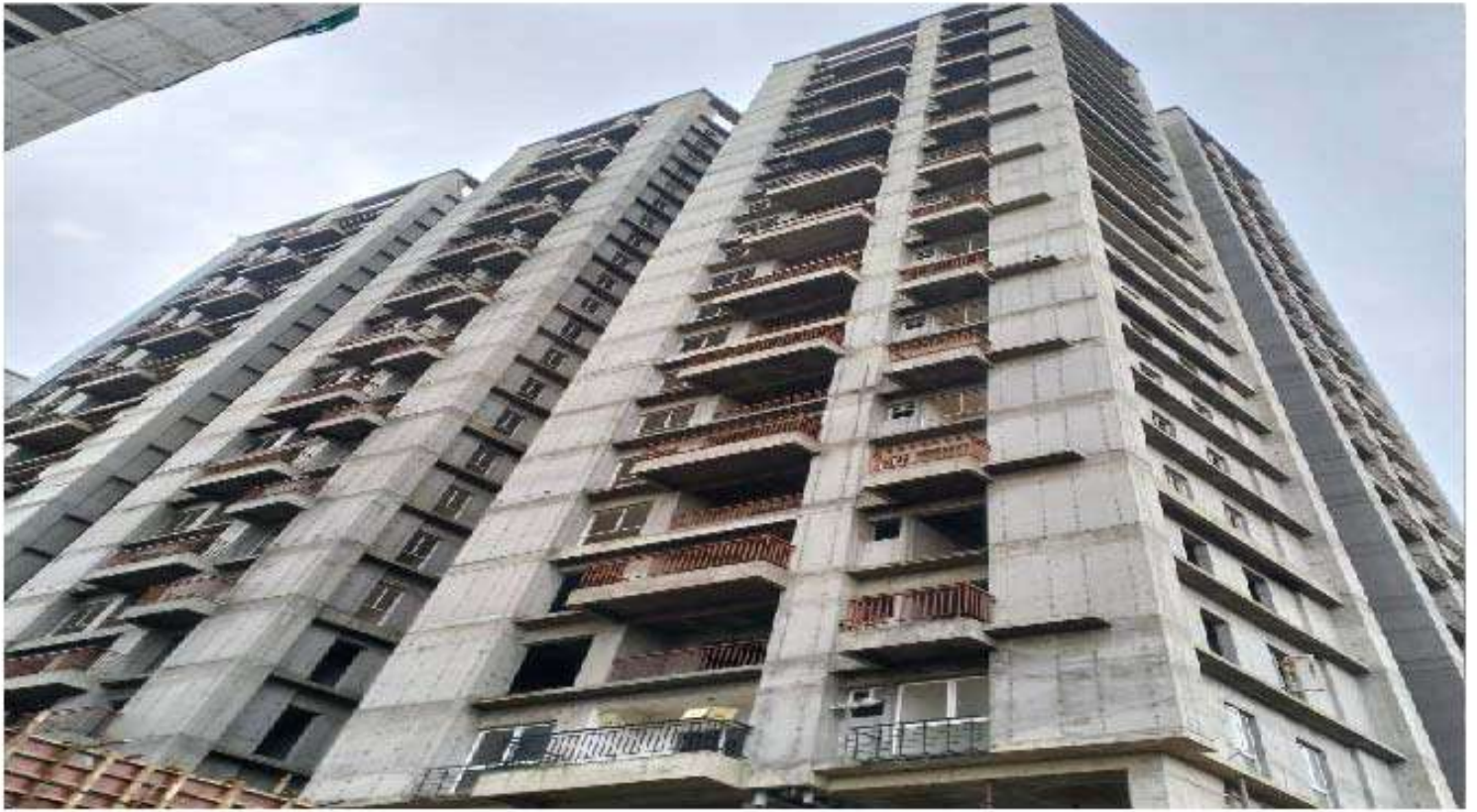
TOWER 2 - EXTERNAL WORK COMPLETED
