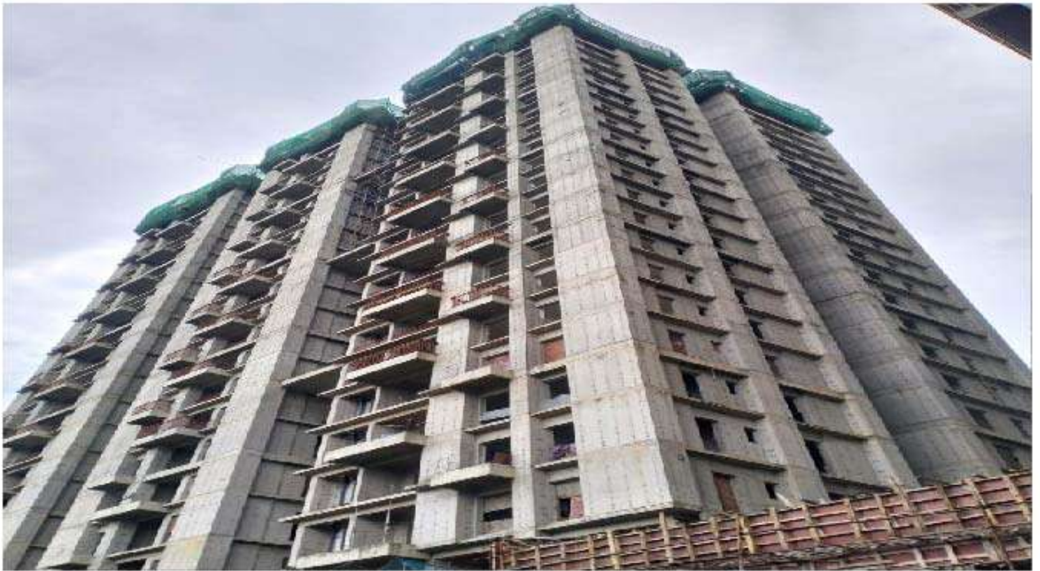
TOWER 1 - SLAB AT ULTIMATE ROOF LEVEL IN PROGRESS
