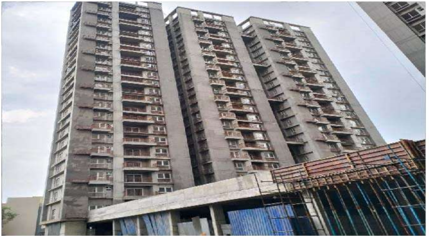
TOWER 3 - EXTERNAL WORK COMPLETED
